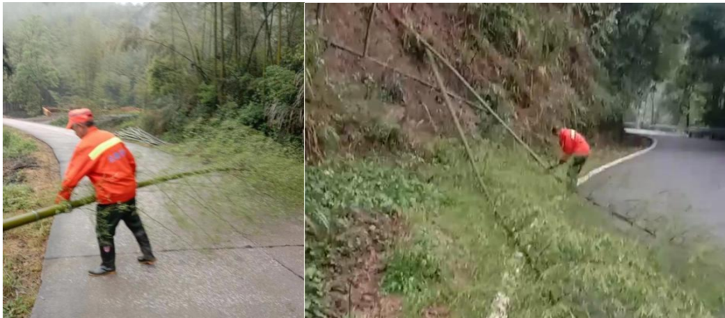
清理倒塌树木
